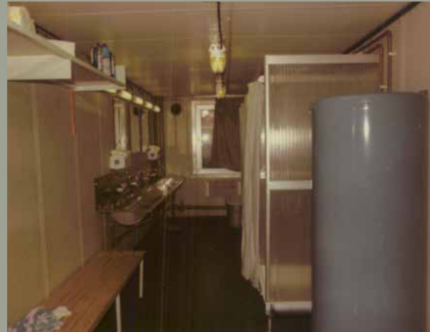
Shower room in the container section on ALK.
